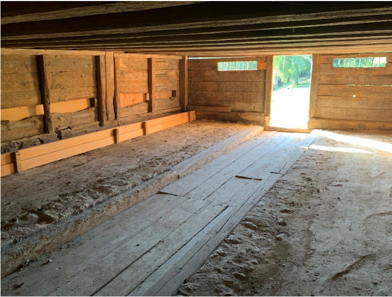
Stallscheune Erdgeschoss links
